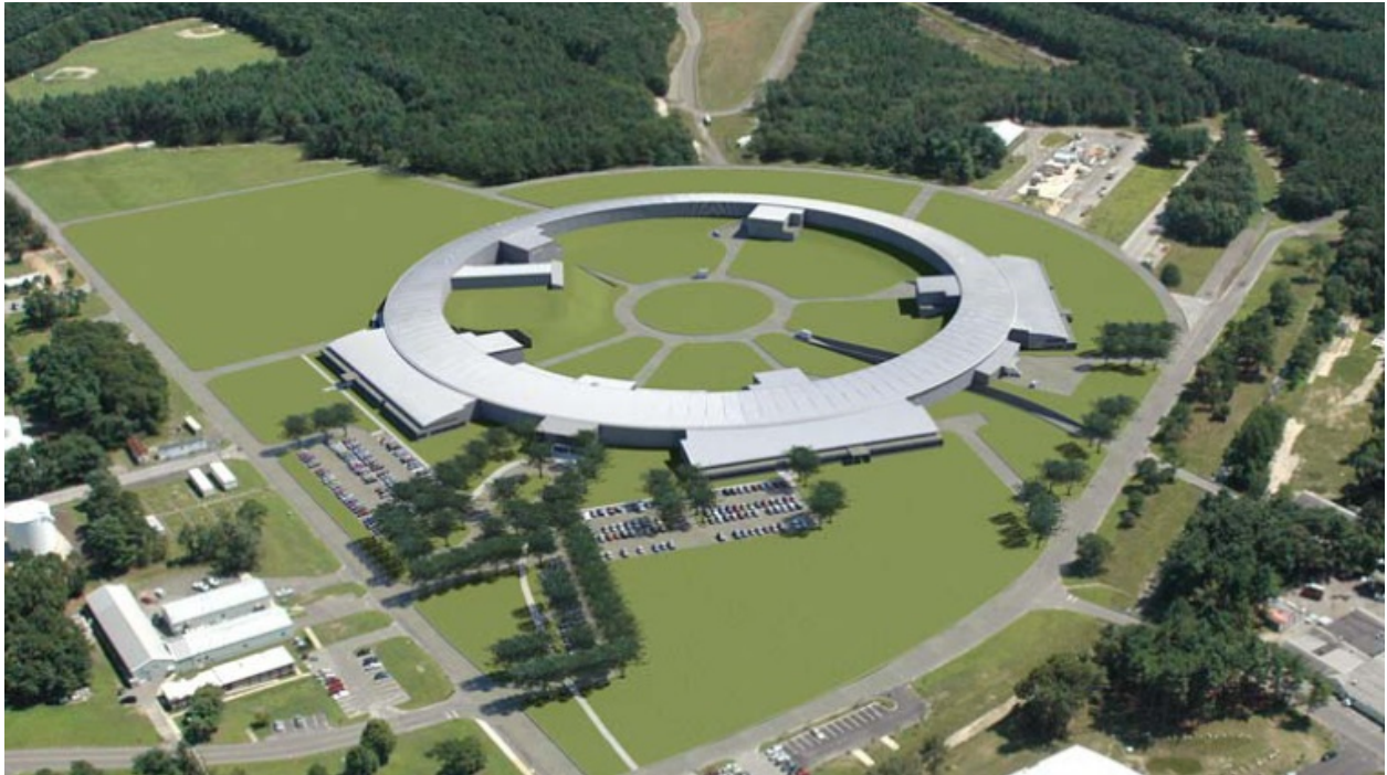
Figure 4: New synchrotron in BNL. The circular building contains a vacuum tunnel where electrons are running with the speed close to the speed of light. The rectangular buildings attached to the circle are the labs where the X-ray experiments are made.
